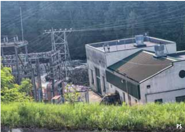
The aging Waltham dam and power station, part of the Upper Pontiac’s hydro grid, needs equipment upgrades to meet growing demand and reduce outages. ent in most of the region, and Bell Canada’s fibre-optic phone service depends on hydro. When the power goes out, so do the landlines. This has left vulnerable residents, including seniors, without any way to call for help during emergencies.
