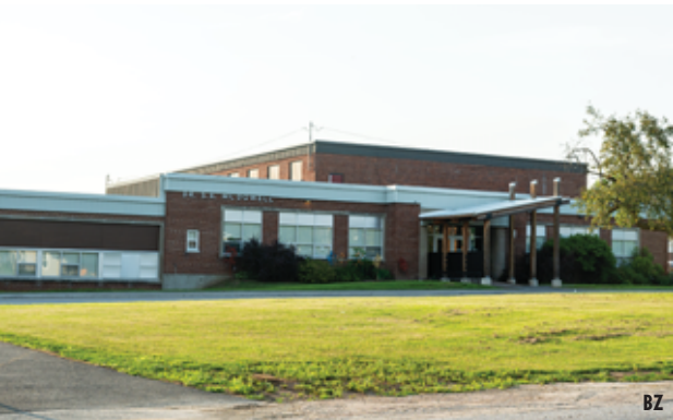
Much-needed renovations have started at Dr. S.E. McDowell Elementary in Shawville. SOPHIE DEMERS LOCAL JOURNALISM INITIATIVE
