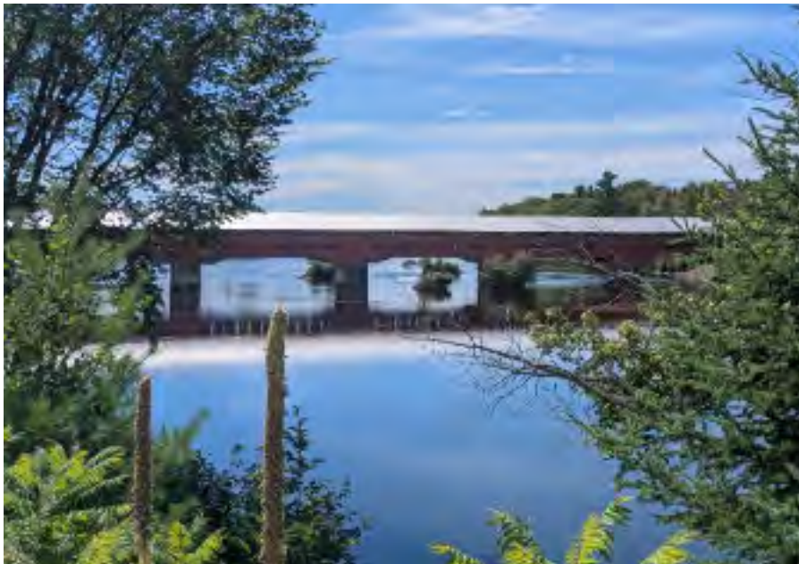
Pont Marchand, Mansfield / Marchand Bridge, Mansfield.
