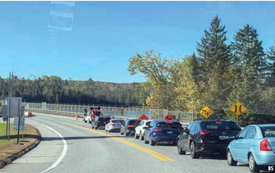
Major repair work has started again on Chenaux Dam bridge. Currently, there is alternating traffic only, with possible complete closures in the future. Read full article on Page 8.
